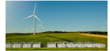
Tesla Powerpack 100MW (megawatts) 2017 South Australia
